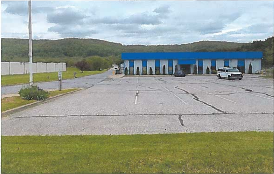
Photo 1: View looking northwest at the existing academy building.
