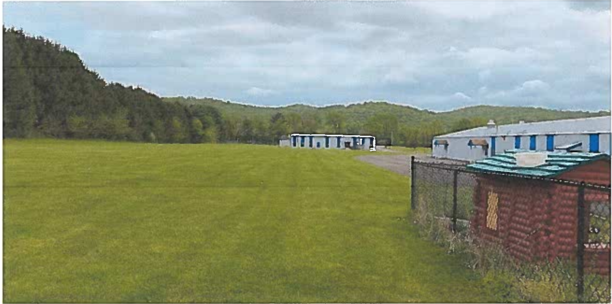
Photo 5: View looking South at the existing academy and warehouse building.
