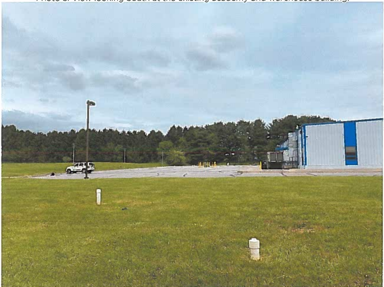
Photo 6: View looking East at the rear side of the existing academy building.
